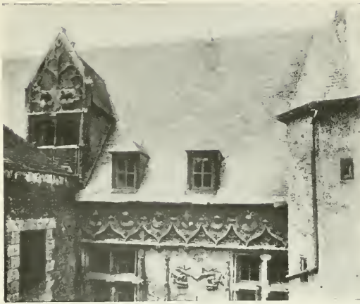
FAÇADE OF THE "BAILLIAGE" (Bailliwick)
